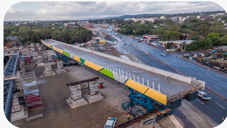
STEEL COMPOSITE BRIDGES
