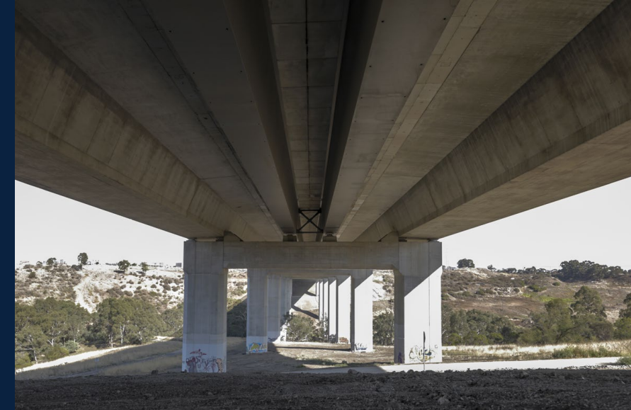
Bridge Widening – An example, Australia
