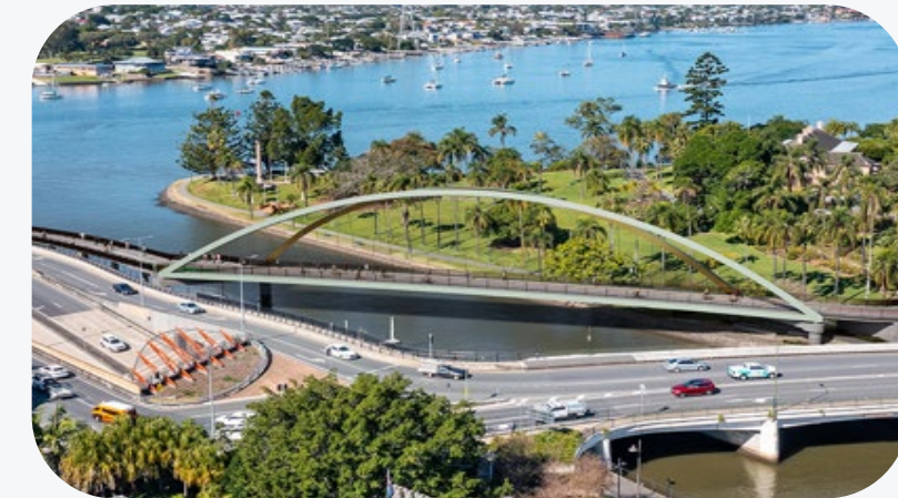
NETWORK ARCHES – PEDESTRIAN BRIDGES
