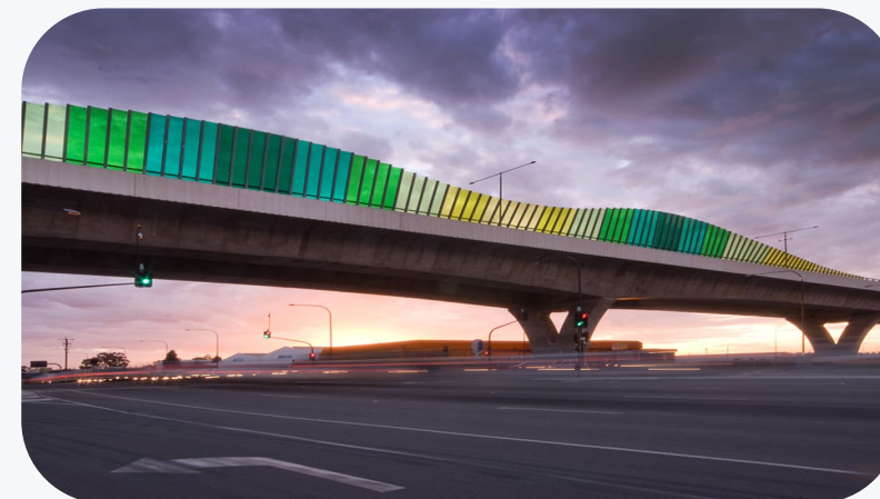
SEGMENTAL PRECAST - BALANCED CANTILEVER
