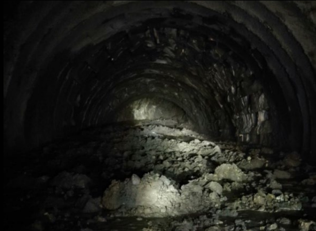
T6+737m Left arch shoulder protruding mud on the face of the tunnel
