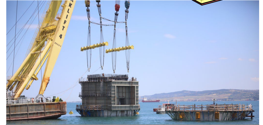
Plinth Form/Rebar Cage Installation
