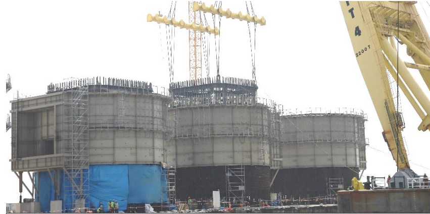
Form/Rebar Cage Pre-Fabrication
