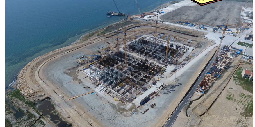
Caisson fabrication in the dry dock
