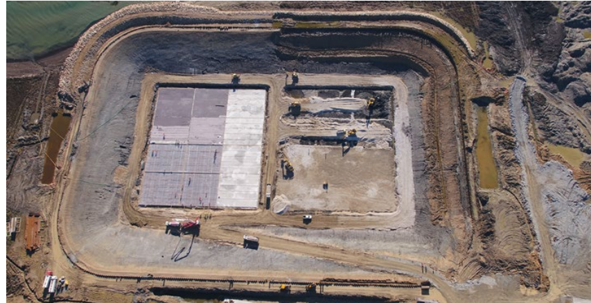
Preparation of dry dock
