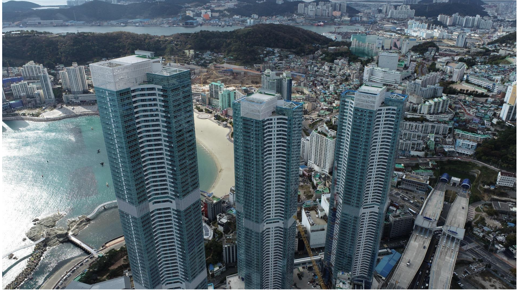
Fin Wall & Belt Wall
